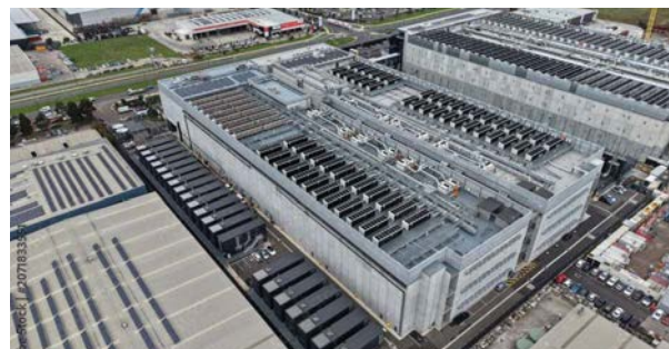
A data center in an industrial district of Melbourne, Australia. Rooftop solar arrays and screened backup generators along the building edge are the kinds of features local standards can require.
