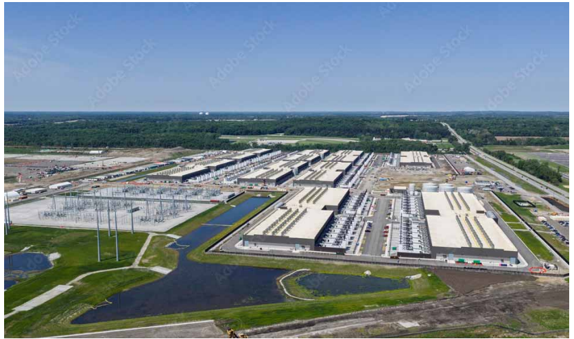
A hyperscale data center campus under construction in Indiana, with its own electrical substation and stormwater ponds. Facilities at this scale can require power and water infrastructure comparable to that of a small city.
