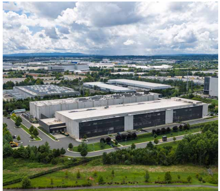
A data center in Ashburn, Virginia, set within an established business park. Vegetative buffers help shield the use from neighboring properties and could lessen the heat-island effects of large-scale data centers.
